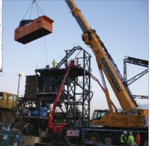
Left. 2.4m x 6m triple deck screen about to be installed in Tarmac Croxden, Stoke on Trent. This unit replaced an Alice Rippl-Flo unit.
